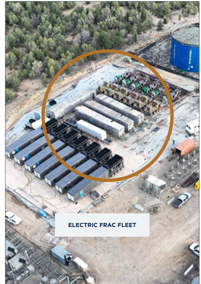
TERRA PAD WITH ELECTRIC FRAC FLEET ON LOCATION
