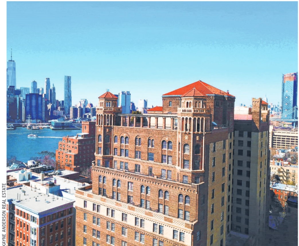
The Watermark at Brooklyn Heights will be converted into a high-end residence for seniors.
